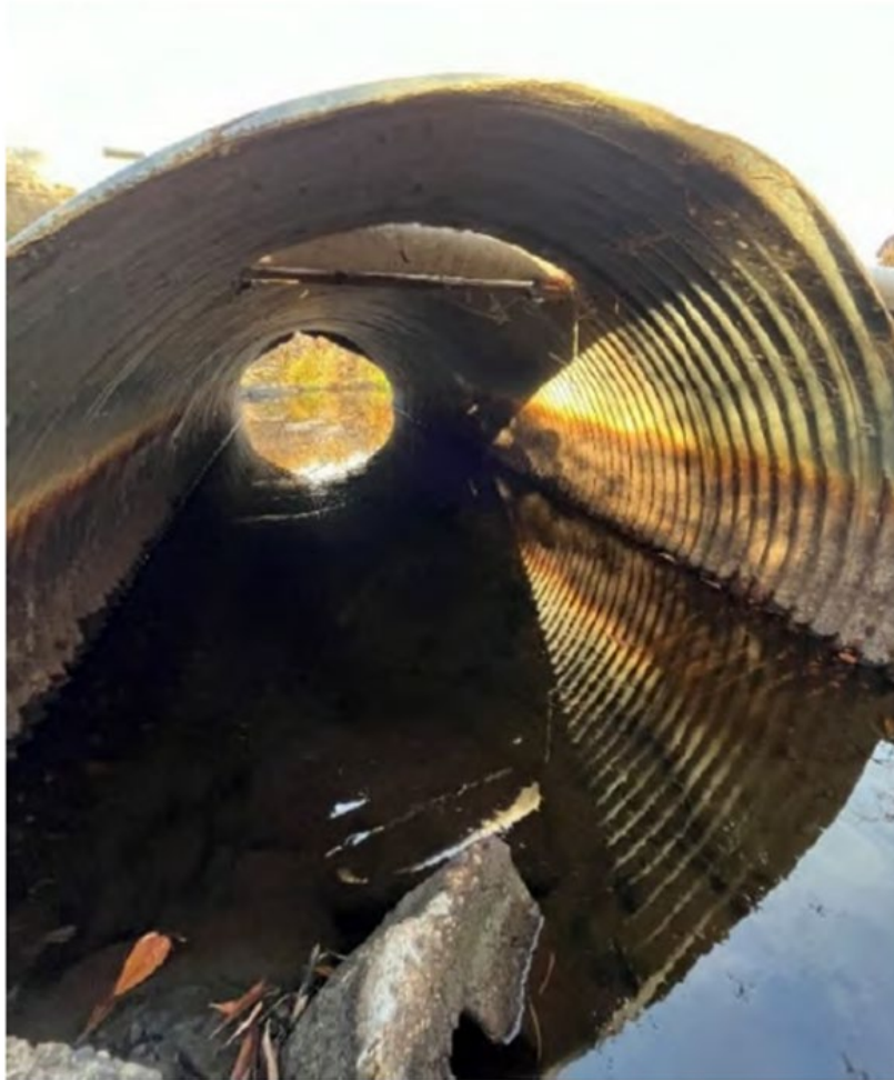
Photo 2: Interior of existing culvert (downstream looking upstream). Irrigation pipe can be seen laying through the crown of the culvert.
