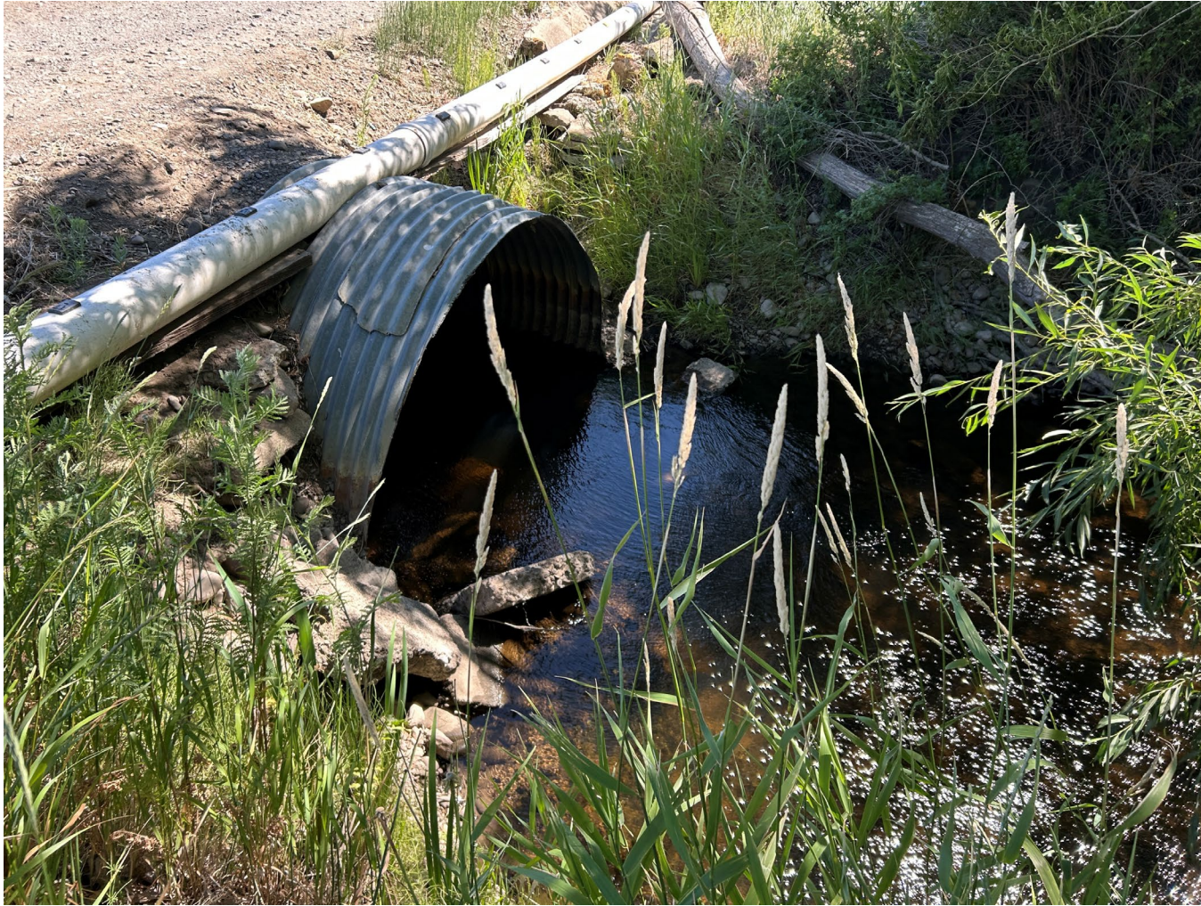
Photo 4: Right bank view of culvert outlet.
