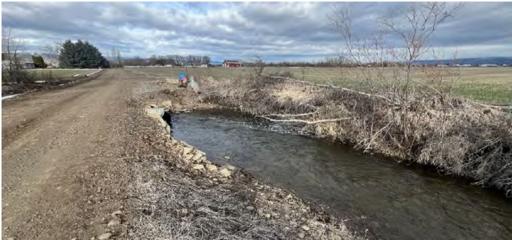
Photo 1: Upstream view of Naneum Creek entering the existing culvert (flowing right to left).
